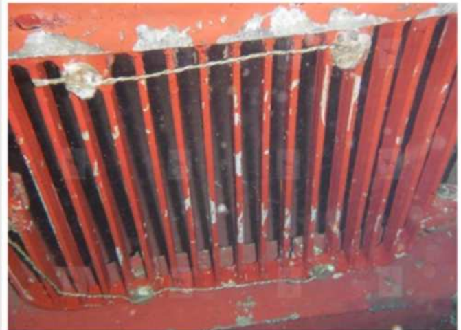
FIRE PUMP GRID POST CLEAN
